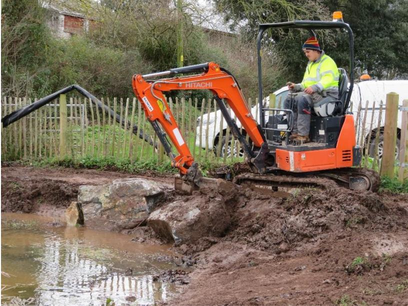
contractors have now widened and stabilised the path by installing some large rocks to form a new edge to the scrape and a gravel finish to the path making it much more accessible to visitors and buggies in particular. The contractors have also regraded the northern edge of the scrape so that there is a more gentle slope, making it easier for any dogs or small children that venture into the mud to climb out again.
